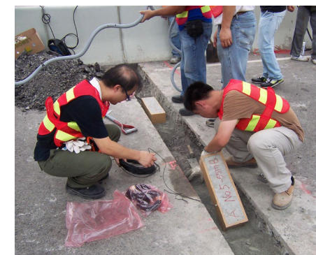
水泥基的壓電傳感器，可監測汽車流量、行車速度和車重。 The cement-based piezoelectric sensors can be used to monitor traffic flow, vehicle speed, and vehicle weight.
