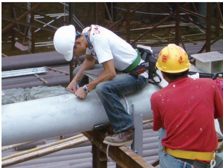
工程研究及檢測中心人員為建築工程進行檢測(圖片由澳大工程研究及檢測中心提供) Centre for Engineering Research and Testing staff are testing a structure (Photo courtesy of the Centre for Engineering Research and Testing of UM)
